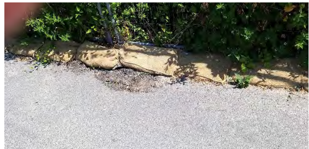
Photo 6. Sandbags placed along the edge of Old Castle Road to prevent water from entering the landslide headscarp. Evidence that the road edge has been affected by subsidence.
