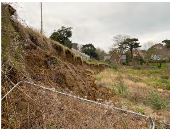
Photo 10. 5th March 2020. Further significant displacement of translational failure and growth of headscarp height. Cliff fall debris from the overstep scarp is visible in the foreground.
