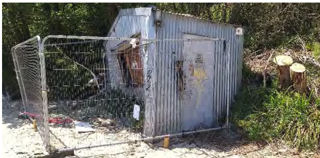
Photo 5. Hut at the southern end of the site has been displaced seaward and twisted by the landslide debris.
